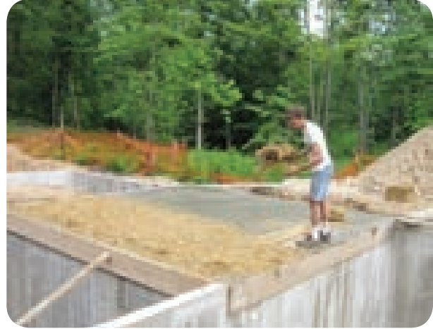
Covering the concrete with wet sand
