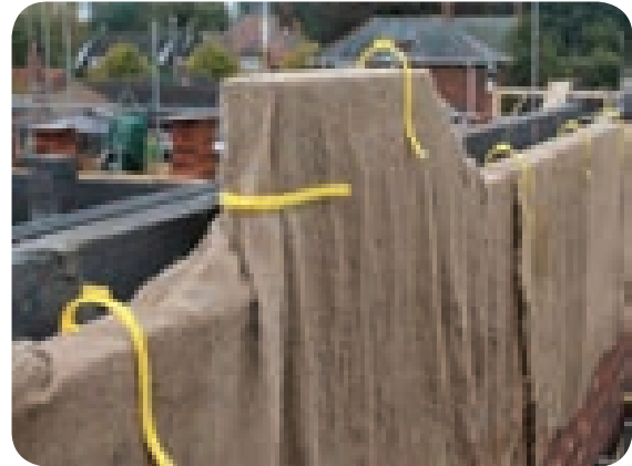
Covering the concrete with, jute bags
