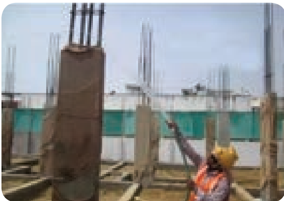
Cured by covering with wet sack
