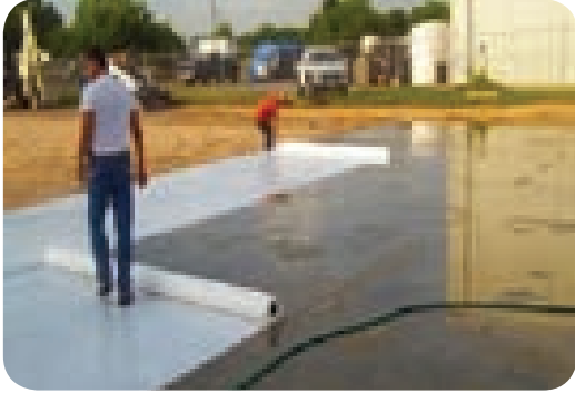
Covering concrete with polythene bags
