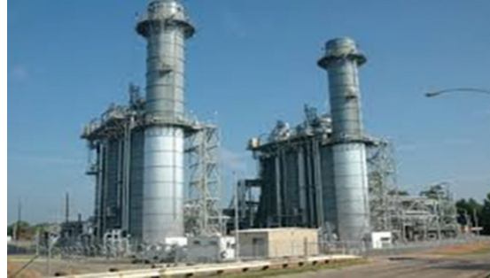
Gas Power Plant
