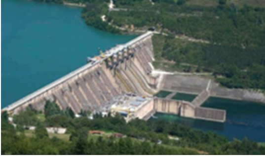
Hydro Power Plant
