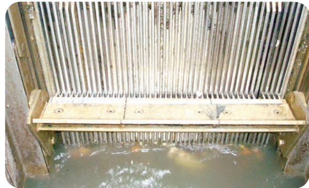
Figure 9.8: Bar Screening in Sewage Treatment
