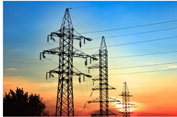
Fig. 1.7 Latticed steel tower
