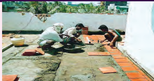
Mason fixing the tiles on the floor.
